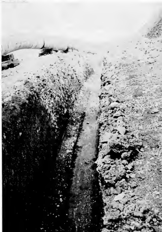
Plate 11. Gas pipeline at crest of Wold scarp: Carstone, Red Chalk and White Chalk. (TF 302772) (Photo by D. N. Robinson)
